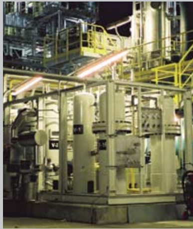
XEBEC H-3100 1000 Nm 3 /hr unit in operation at a European oil refinery.
