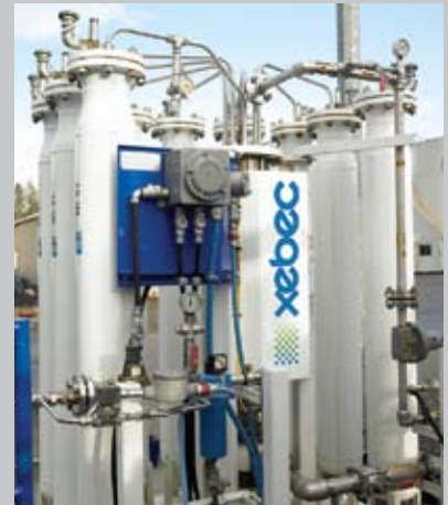
XEBEC H-3200 recovering hydrogen from off-gas at a chemical plant in North America.
