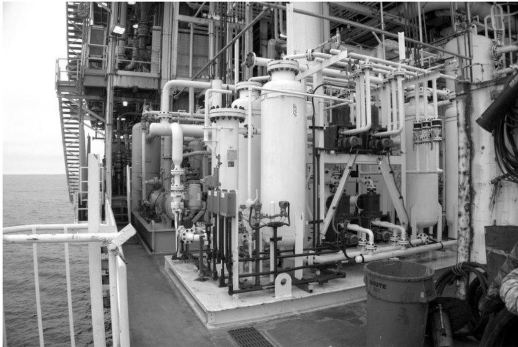
**Figure 6.** Photograph of Entire Xebec Rotary-Valve, Fast-Cycle Pressure-Swing Adsorption Unit On-Board Platform Gail (note – above rotary valves)
